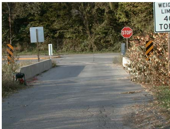
Figure 2.8. Roadway view of Bridge #3.
