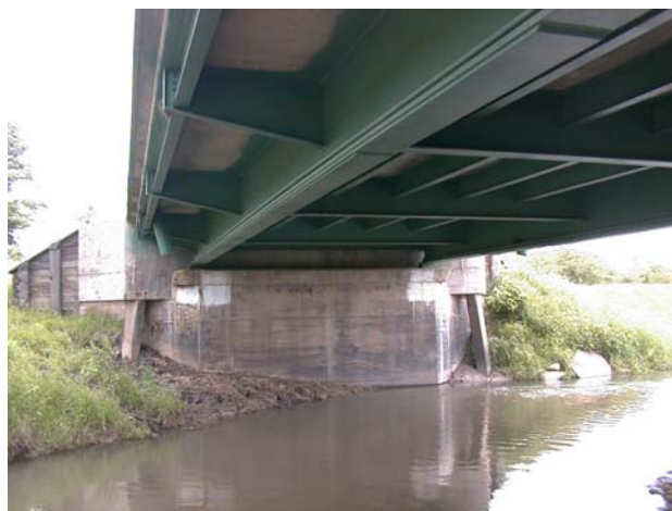
Figure 3.1. Photograph of the main girders of bridge one.
