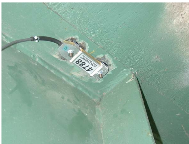
Figure 4.2. A BDI Intelliducer in use on a steel girder.
