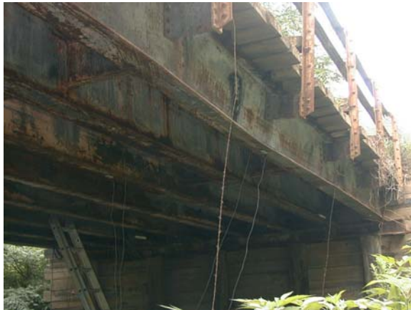
Figure 2.2. Photograph of the bridge railing on Bridge #1.
