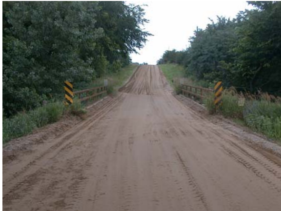
Figure 2.1. Photograph of the south abutment and superstructure of Bridge #1.
